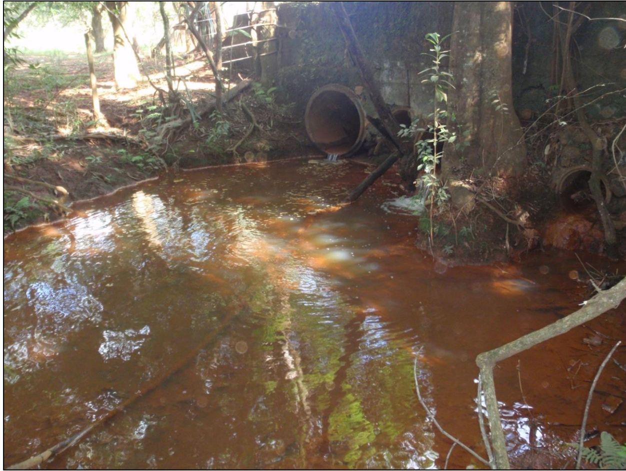
Red-brown color in discharge from dam drainage pipes after water treatment Morro do Ouro Mine, Paracatu, Minas Gerais, Brazil
